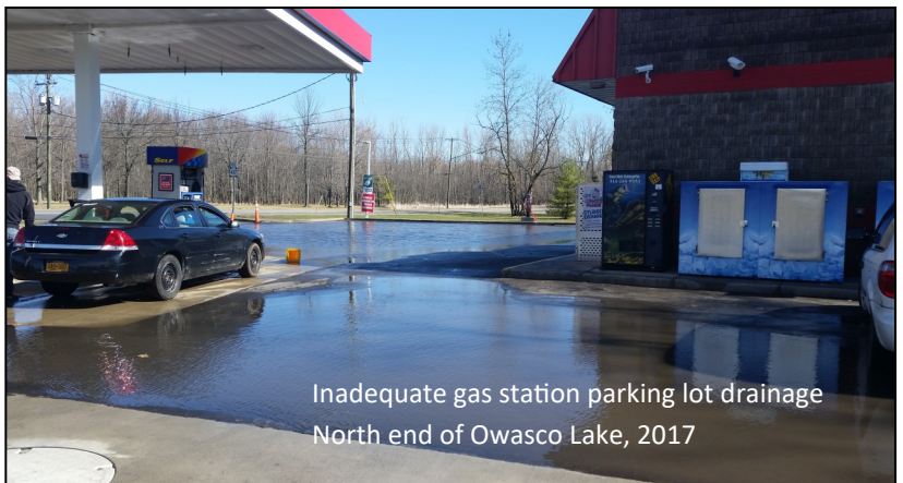
Ineffective stormwater practice installation Sucker Brook subwatershed, 2017
