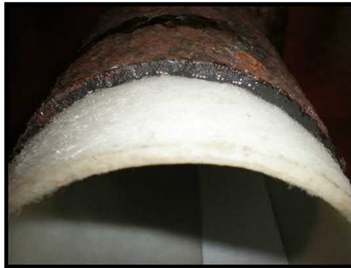
CIPP Liner cured within ductile iron “host” pipe
