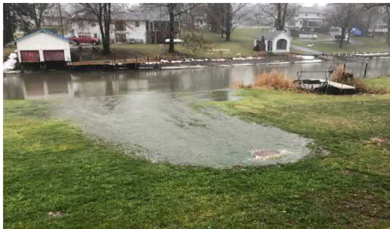
Manhole along Owasco Interceptor Overflowing into Owasco Outlet
