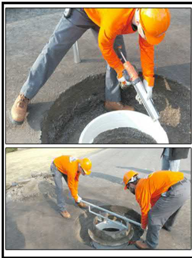
Manhole Riser Ring (Source: Brenneman Excavating Inc.)
